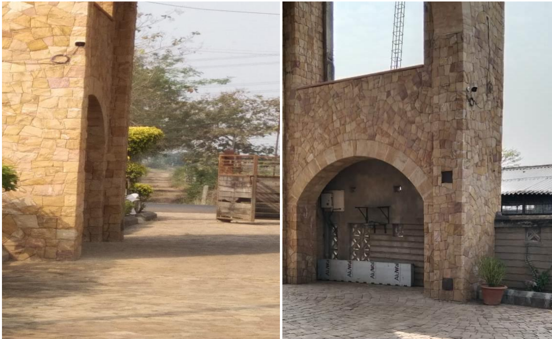
‘CCTV Cameras at Entrance’
