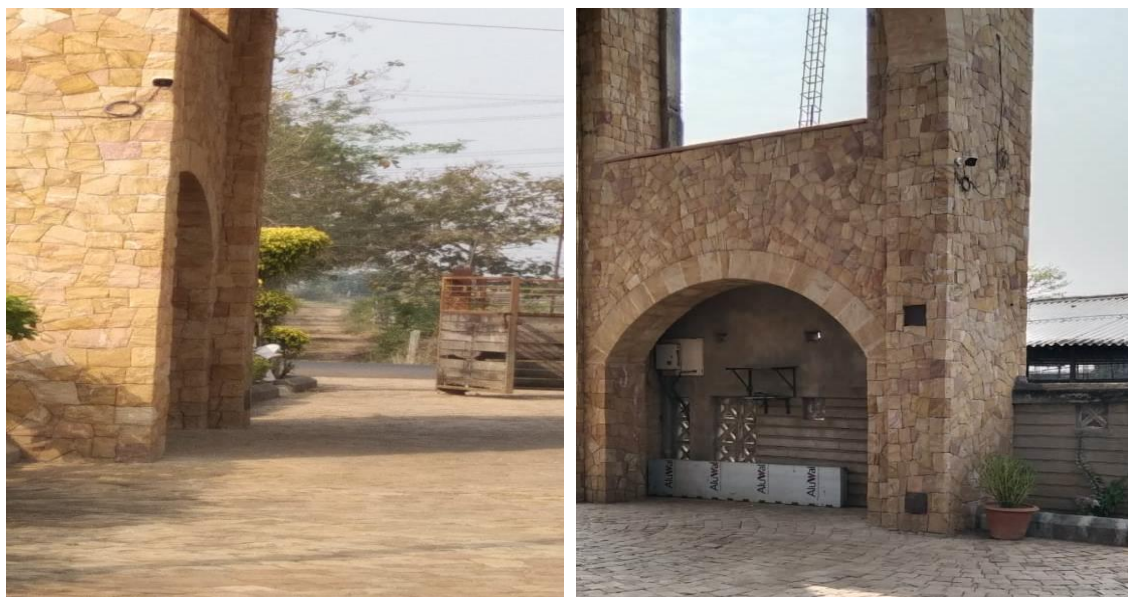
'CCTV Cameras at Entrance'
