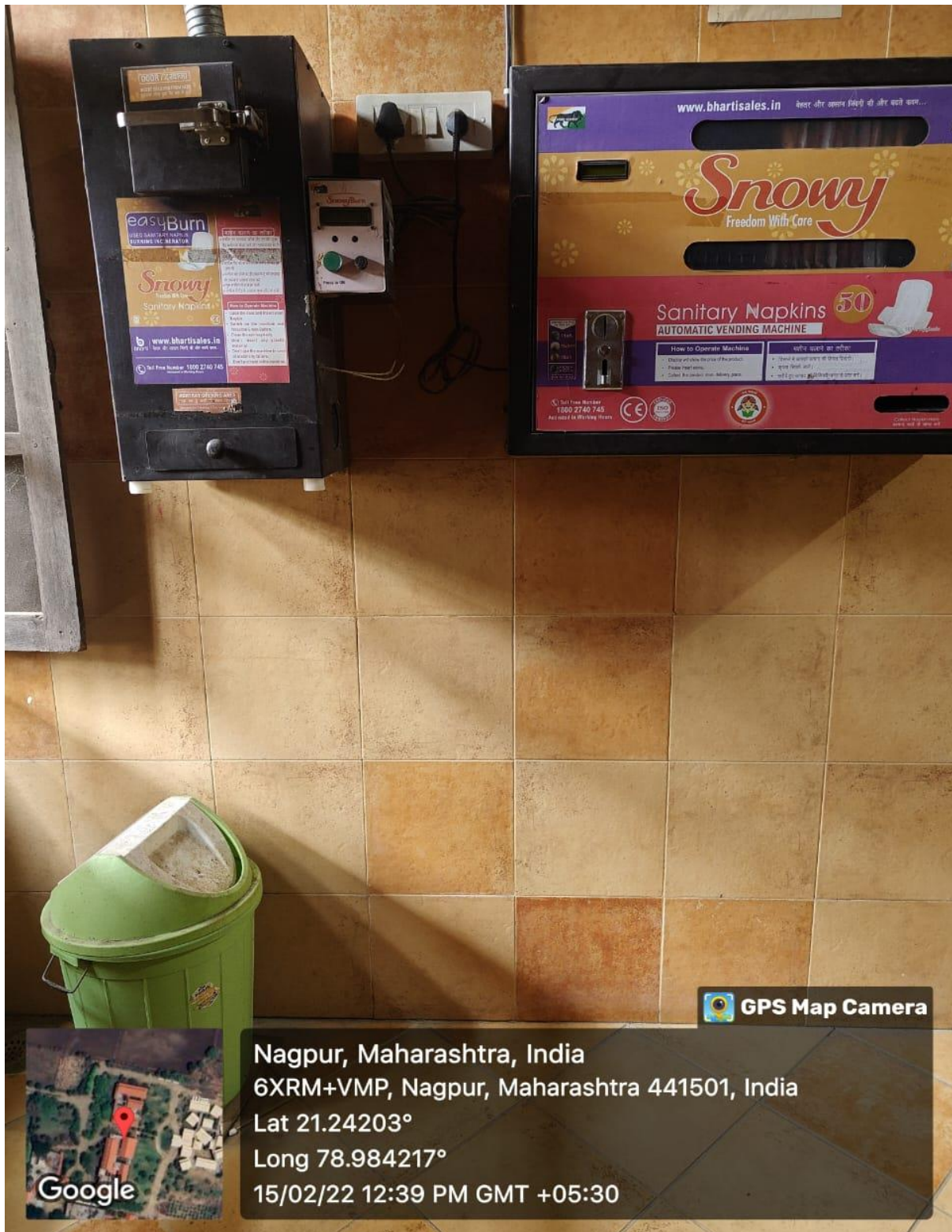
Sanitary pads vending machine & Incinerator
