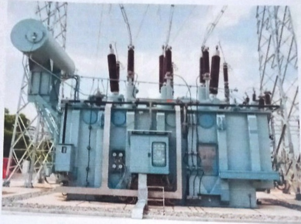
Fig 5.1: Generating Transformer
