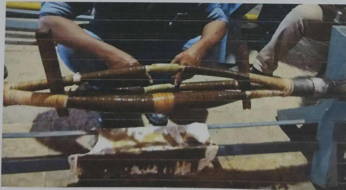
JOINTING OF PILC CABLES at TIPL Workshop
