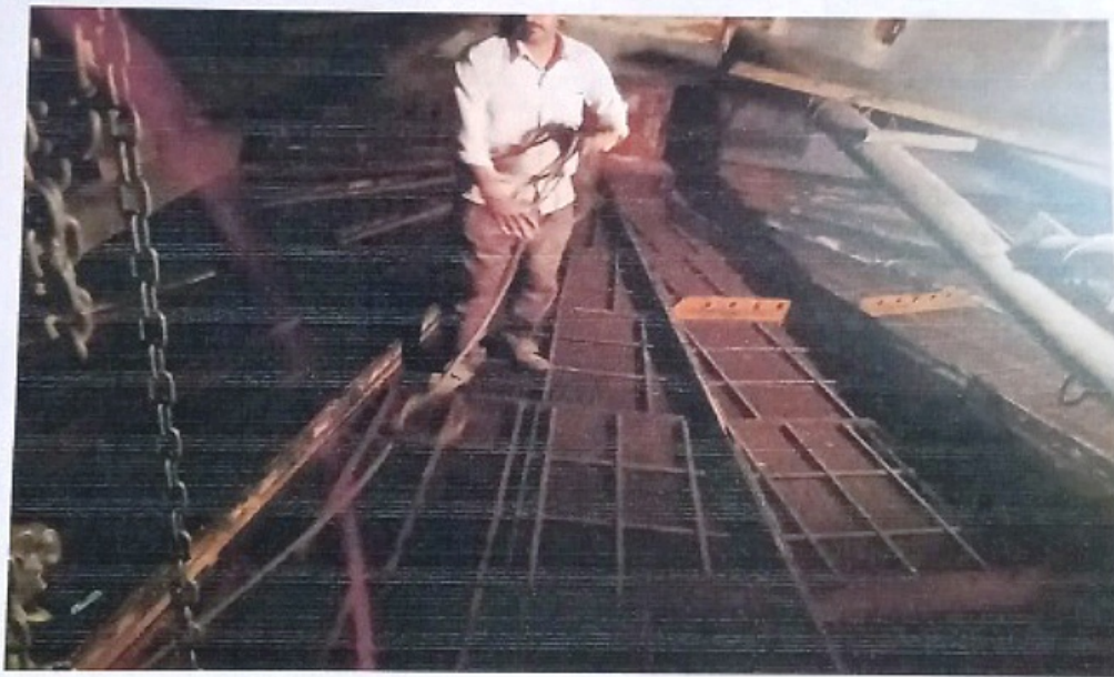
Fig 3.11: Air Preheater
